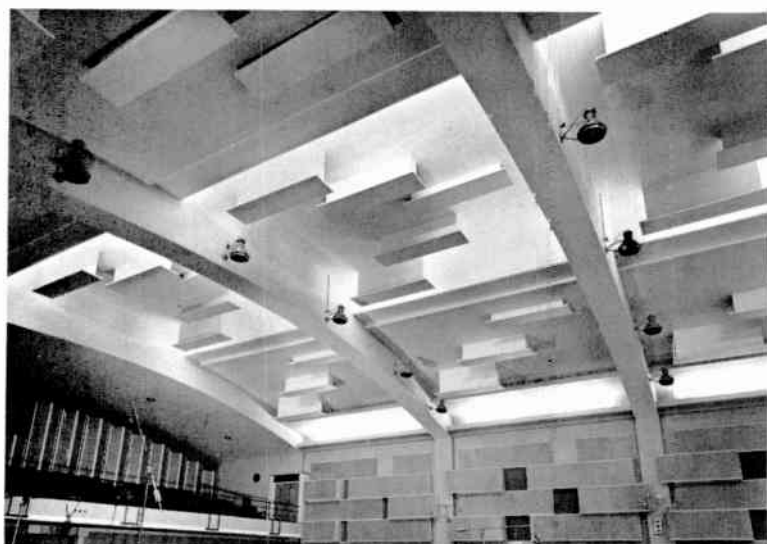
FIG. C/17. Maida Vale Studio 1. Excellent view of ceiling showing variation in size and shape of scattering elements. Note also boxes on side walls which act as acoustic absorbers and diffusers, with special treatment of wall behind small balcony where audience is accommodated.
