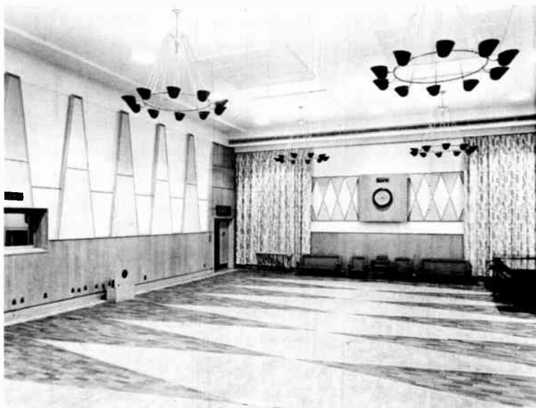
FIG. C/15. Maida Vale Studio 3, showing acoustic curtains in background and absorbent panels of special shape on side walls and ceiling. The wooden panelling near the floor provides low frequency absorption. Note baffle mounted talk-back speaker on the left.
